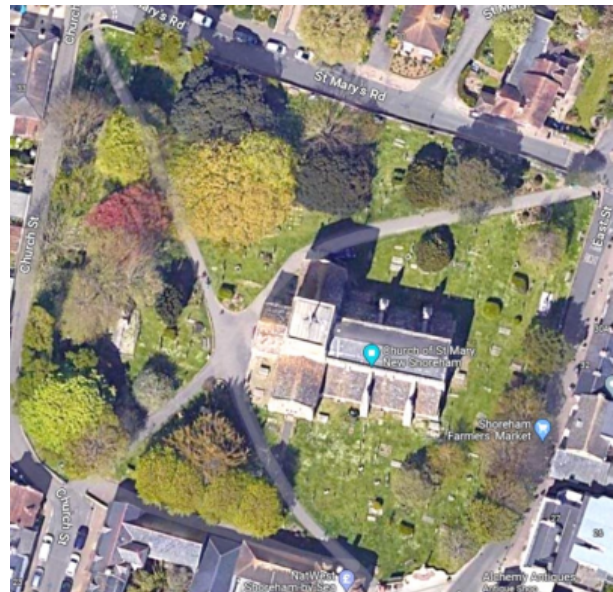
St Mary's situated in the centre of the town
